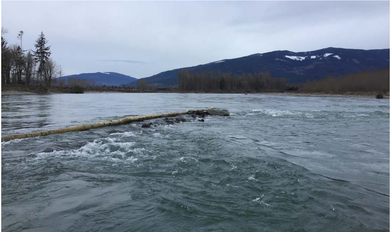
Figure 4. Skiyou rock, view looking upstream near the center of the channel. Log raked against the rock illustrates the 40 degree angle alignment (0 being upstream) that forms a bend-way weir that sets up a grade line perpendicular to its alignment – directing flow away from right bank. This is the eastern edge of the intact rock segments (March 10, 2020).
