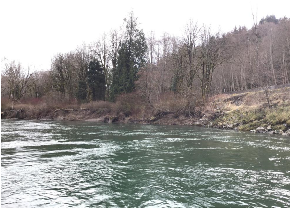
Figure 5. Left bank along the South Skagit Highway, view looking in the upstream direction. Riprap is visible in the foreground of the photo. Note eroding bank upstream where riprap is not present.
