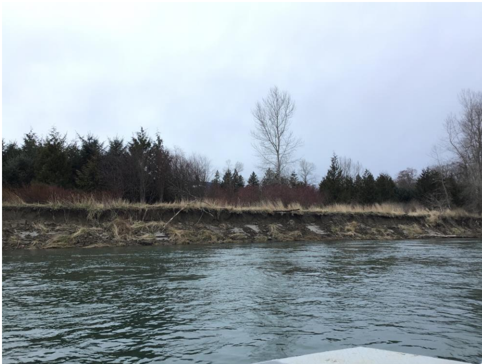
Figure 8. Right bank of the Skagit River immediately downstream of the Skiyou Slough inlet. Flow direction is from right to left of photo. Active sloughing of the streambank indicates undermining of the bank toe.
