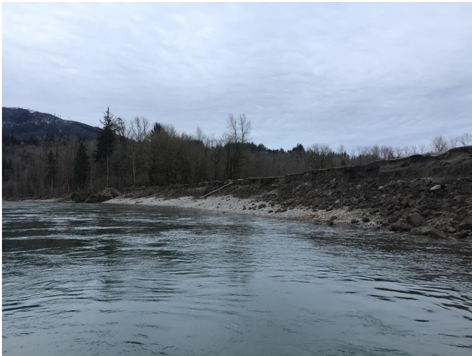
Figure 10. Right bank of the Skagit River immediately along the Benson parcel and evidence of active erosion, located upstream of Skiyou rock. Flow direction is from right to left of photo.
